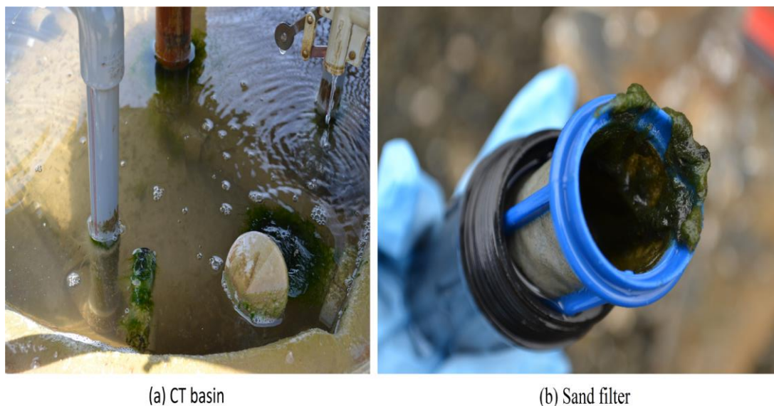
Fig. S1. (a) Algal growth in CT basin and (b) suspended algae captured in sand filter.
